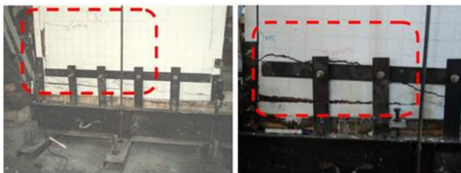
a. Flexural crack which occurred in the plastered-bamboo wall with wiremesh bracing
