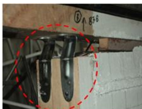
a. The upper right joint was almost dislodged (panel without bracing)
